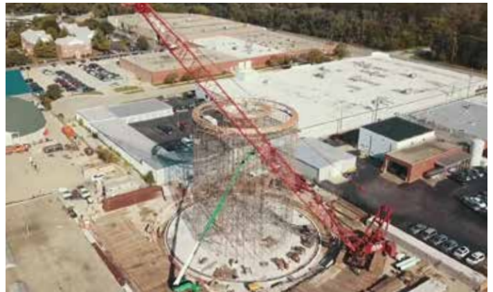
Seven-million-gallon water reservoir under construction in Morton Grove, courtesy of the Morton Grove-Niles Water Commission
