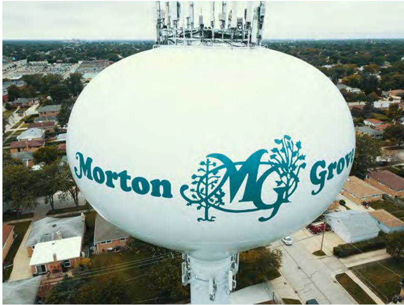
North Pumping Station elevated water tank - The capacity of the North Pumping Station elevated water tank is 750,000 gallons.
