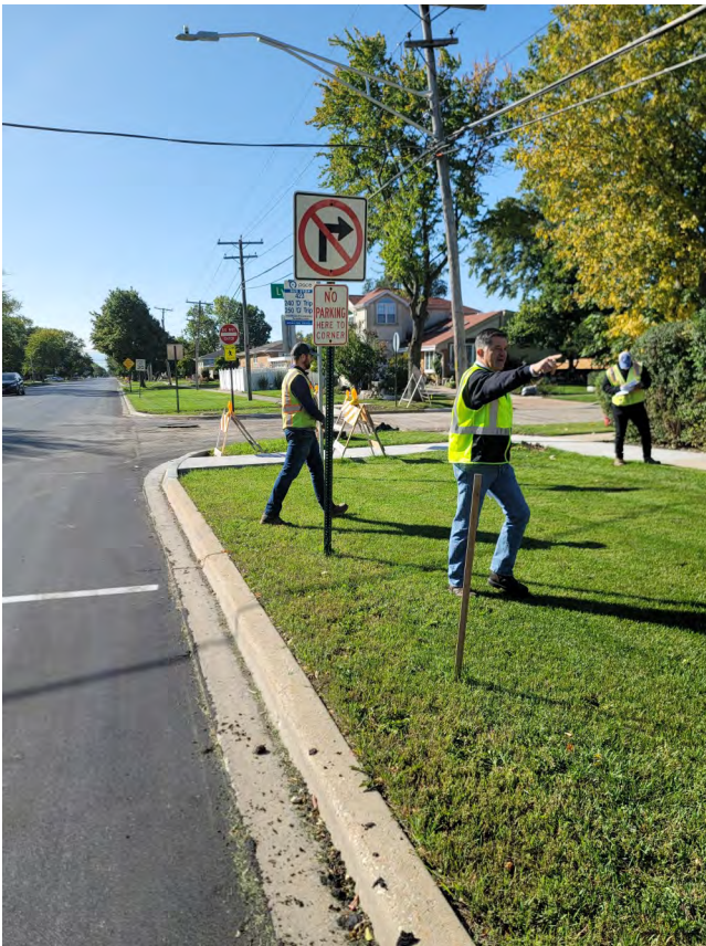
Village engineering personnel & consultants reviewing project closeout at the Harlem Avenue and Shermer Road pavement overlay
