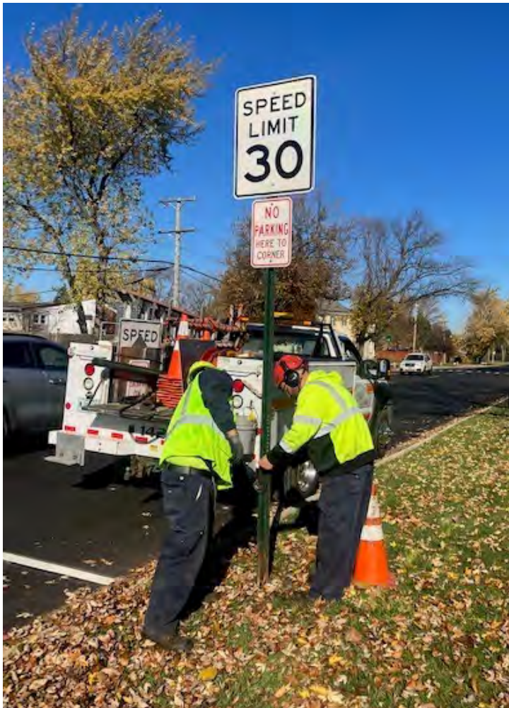
Street Sign and Pole Installation at Harlem Avenue and Emerson - Installation of new signage to align with pavement markings was completed by the Streets Division after the roadway was re-paved by the Illinois Department of Transportation (IDOT).
