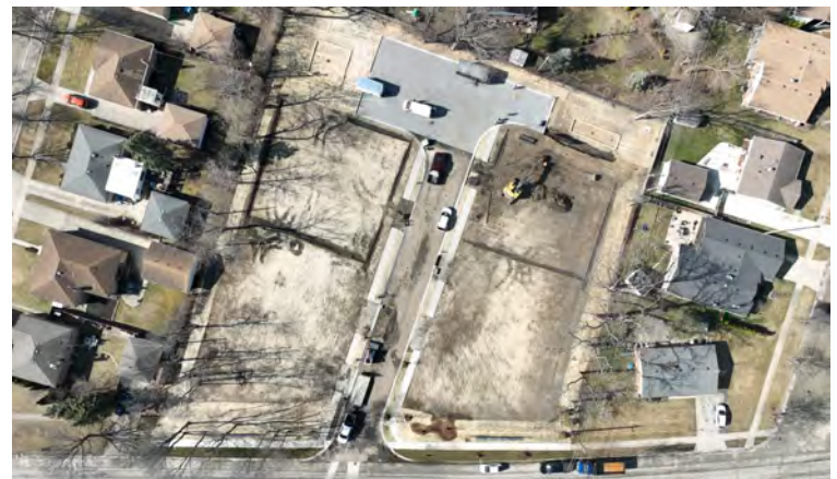
New Ponto Court Subdivision (aerial view taken after utility connections and site work)
