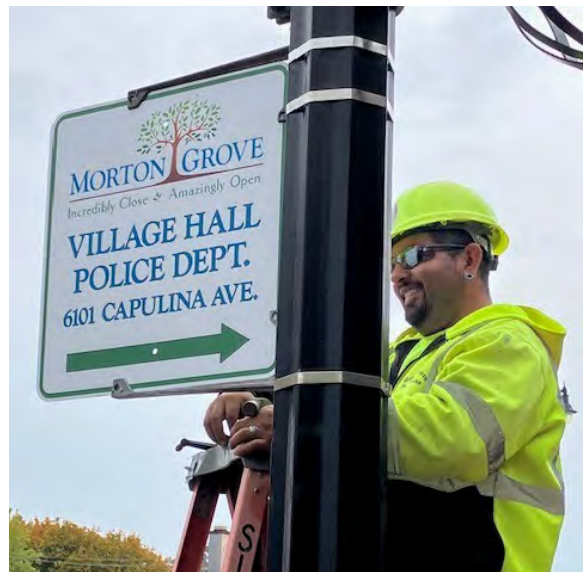
Village Informational Sign Installation at Dempster Street and School Street
