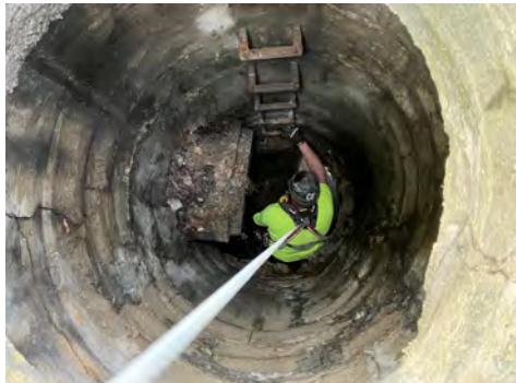
Storm Sewer Entry for Sewer Televising Prior to Village-Contracted Sewer Lining - When Sewer Division personnel enter the sewer manhole (a confined space), they are required to connect into safety harness cables (as seen above). The Envirosight ROVER X sewer televising camera is placed into the storm sewer pipe for evaluation prior to completion of sewer lining by the Village-contracted company.
