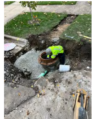
Catch Basin Replacement on Parkside Avenue - Excavation of the area was completed to access and deconstruct the deteriorated catch basin. The former catch basin was removed and the new pre-cast cement catch basin was placed. Manhole blocks were then used to build up the catch basin to street level. In 2023, eight (8) catch basins were replaced.
