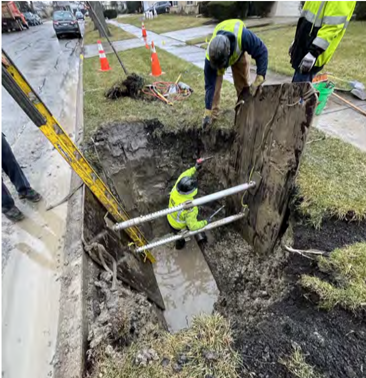
Water Main Break Repair on Merrill Avenue - After excavation, Water Division personnel set up shoring within the hole to protect crew members from trench collapse as they worked to repair the water main break.
