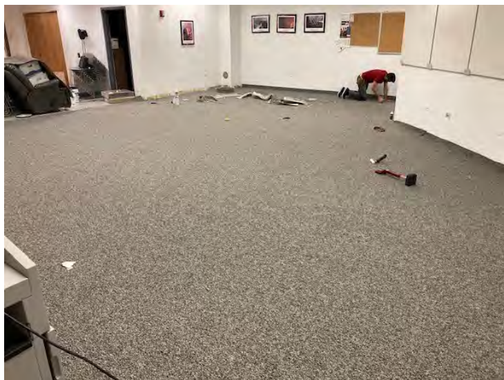
Fire Station 4 Carpet Installation
