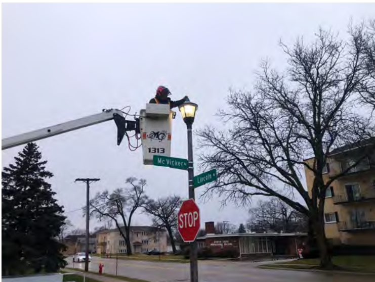
Village Light Pole Photocell Repair at Lincoln Avenue and McVicker Avenue - The photocell within the street light detects light and darkness, causing the light to remain off during the day and turn on at night.
