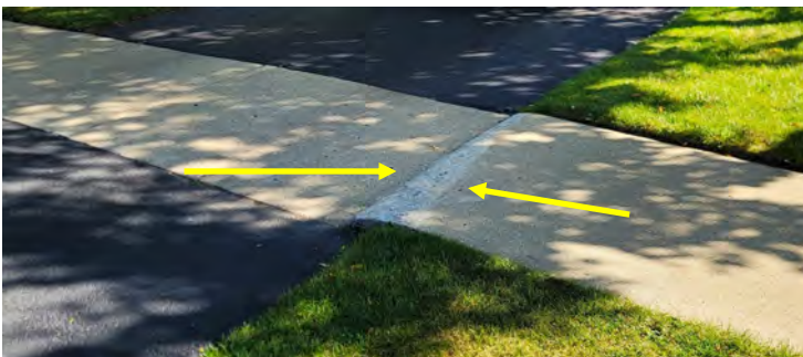
Sidewalk Concrete Saw Cutting
