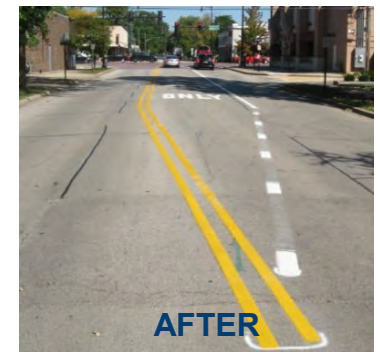
Thermoplastic Pavement Marking at Austin Avenue and Dempster Street
