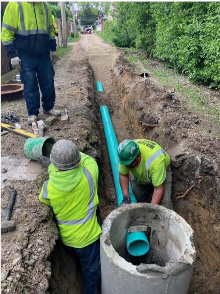
Alley Storm Sewer Pipe Replacement (between Washington Street and Madison Street east of Central Avenue) - Storm sewer pipe replacement was completed in order to improve alley drainage.
