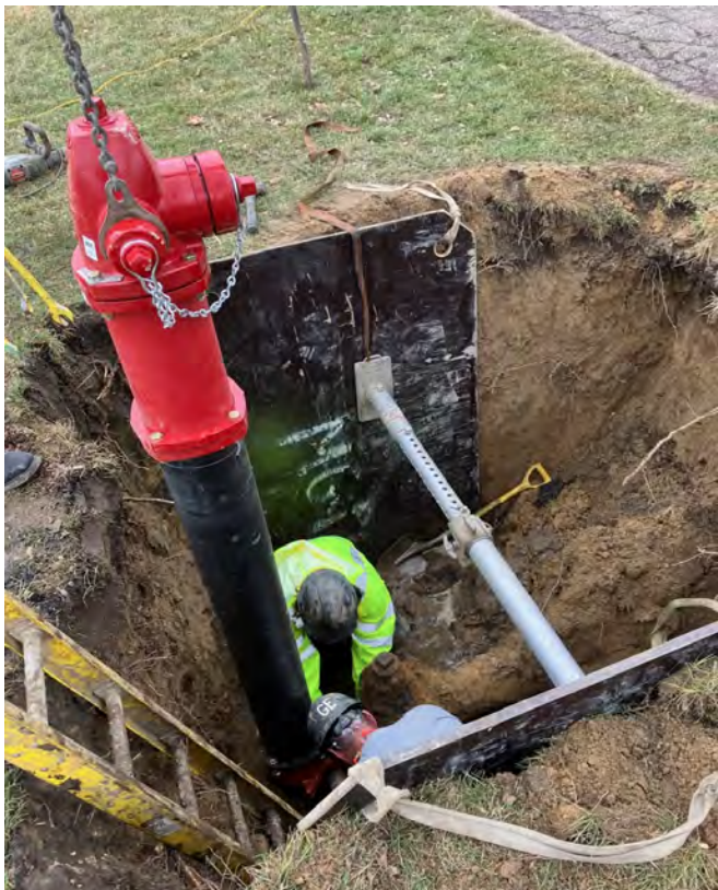
Hydrant Replacement on Reba Court - Excavation was completed to replace a 1928 A.P. Smith fire hydrant with a new Waterous Pacer fire hydrant. A backhoe (not pictured) is used to lower the hydrant down to be connected to the water main.
