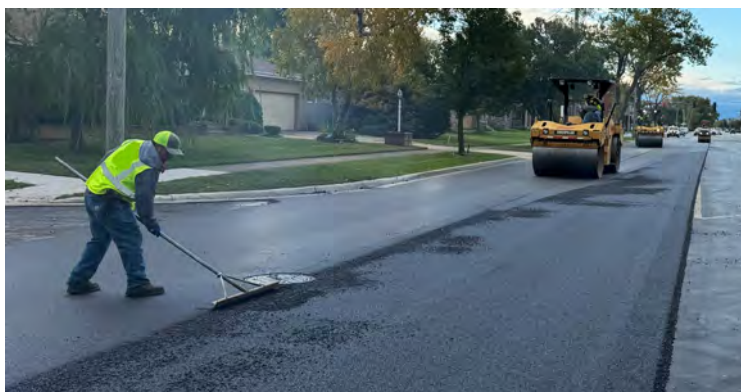
2023 Street Patching Program - Installation of Hot Mix Asphalt
