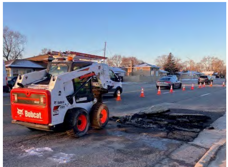
Hot Mix Asphalt Utility Pavement Repair at Dempster Street and Osceola Avenue - The Bobcat breaker was used to remove the temporary cold mix asphalt patch to complete permanent pavement repair with hot mix asphalt.
