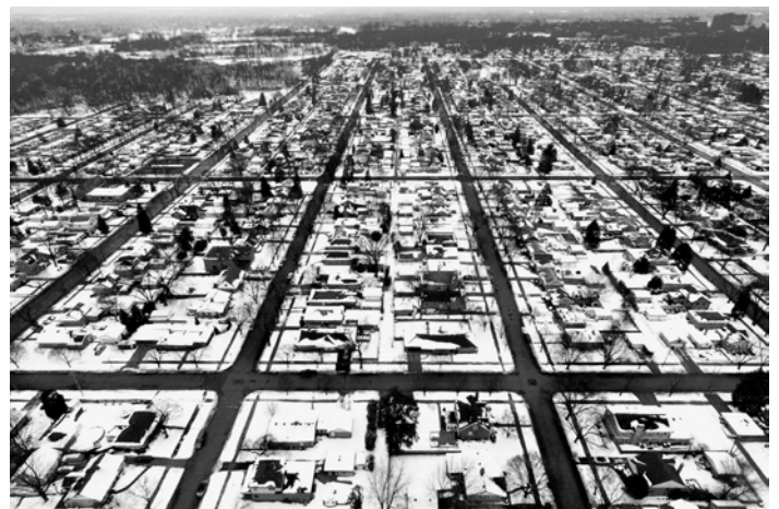
Annual programs and projects developed by the Engineering Division maintain or expand infrastructure systems within the Village
