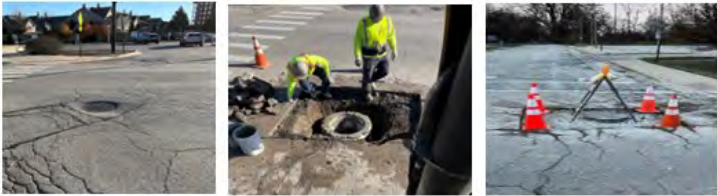
Sanitary Sewer Manhole Rebuilt at Chestnut Street and Lehigh Avenue - Sewer manholes, which allow physical access to the sewer system, require rebuilding due to deterioration over time. The manhole rebuilding process from start to finish is pictured above.
