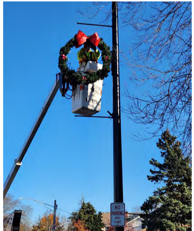
Seasonal Decoration Installation Throughout the Village - Forestry Division personnel utilize the bucket truck in order to complete installation of seasonal decorations, banners, and flags as well as tree trimming and street light photocell repair.
