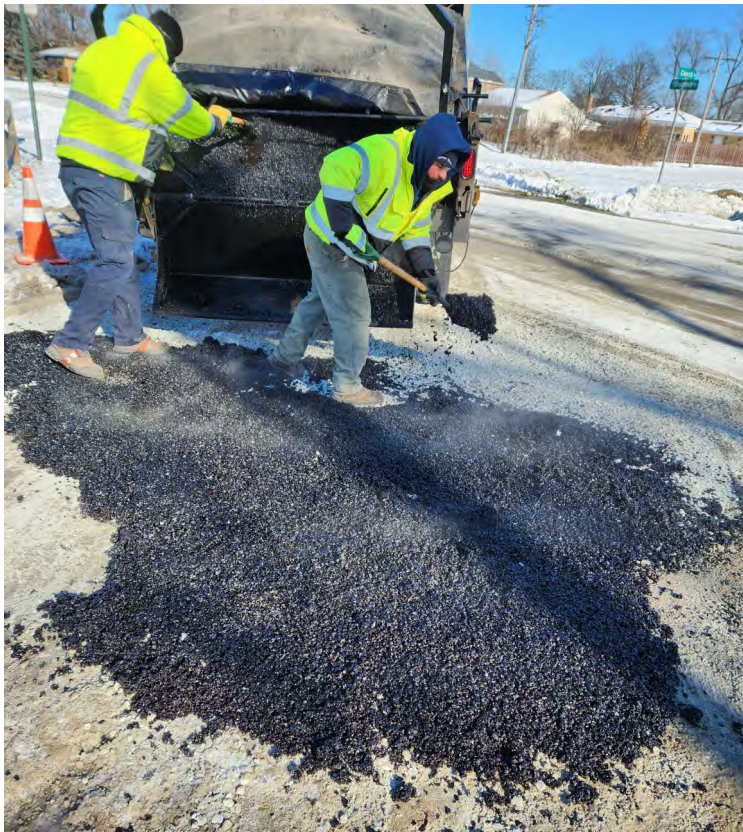
UPM Cold Mix Asphalt Utility Pavement Repair at Church Street and Osceola Avenue - Streets Division personnel placed a temporary cold mix asphalt patch until permanent pavement repair could be completed in Spring 2024.
