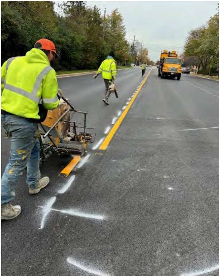
Arterial Street Improvement Program Thermoplastic Pavement Marking
