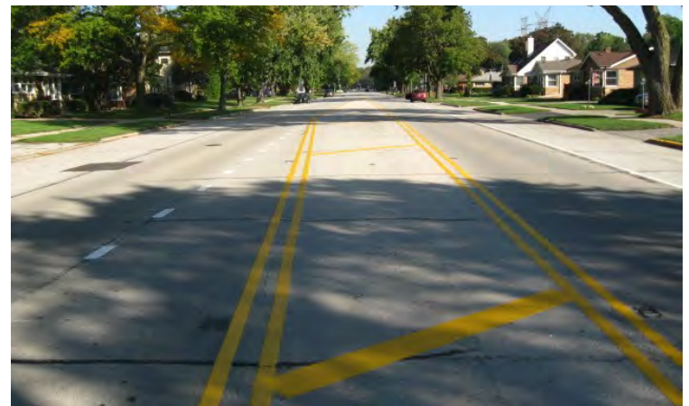
Thermoplastic Pavement Marking at Central Avenue and Church Street (AFTER)
