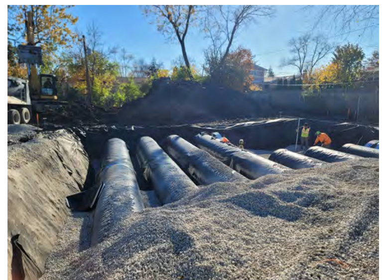
Installation of Underground Stormwater Detention Structures at Ponto Subdivision
