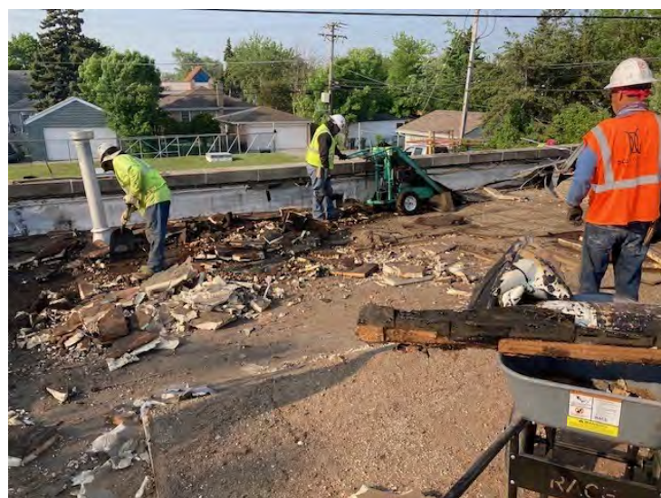
North Pumping Station Roof Replacement
