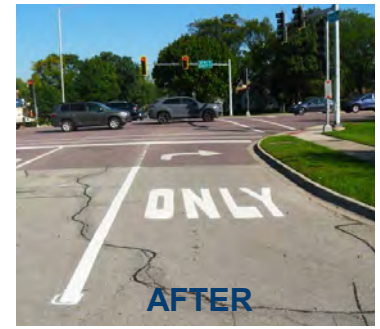
Thermoplastic Pavement Marking at Central Avenue and Dempster Street
