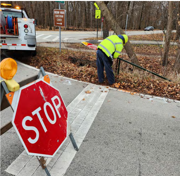
Stop Sign Installation at Austin Avenue and Beckwith Road - Streets Division personnel completed stop sign installation to replace the previous damaged pole and sign. A temporary stop sign was placed (as seen in the foreground) to ensure traffic safety during sign installation.
